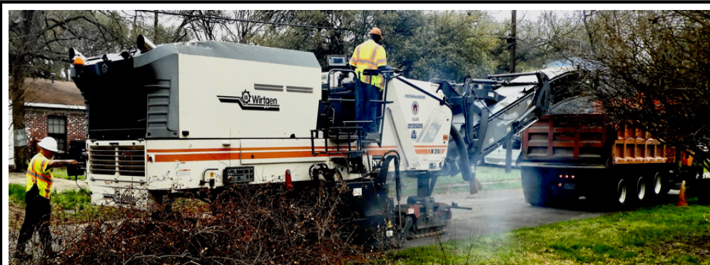
This is the monster machinery precisely scraping/grinding about 2" off the surface of Whitewing
